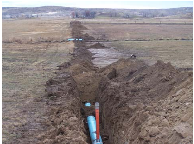
After: 2,800 feet of buried mainline for sprinklers.
