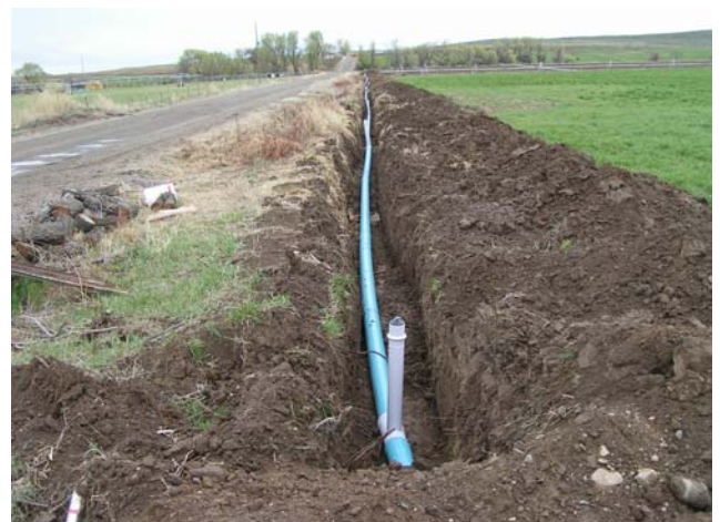
After: 2,700 feet of buried mainline and sprinklers.
